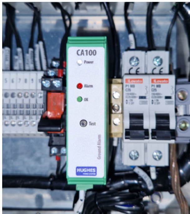
Installation in the motor drive cabinet
